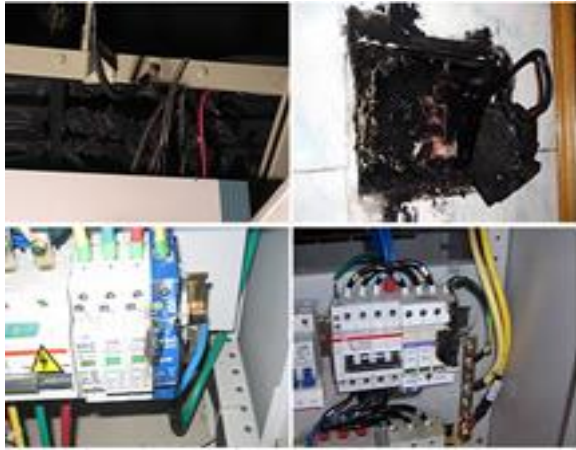
Fig.1. Photos of SPD failure and burn in fields
